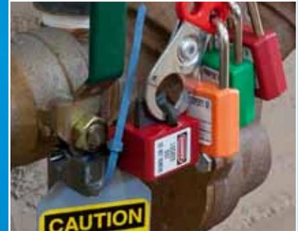
S3068 locking out valve with 410s and S4051MT tag
